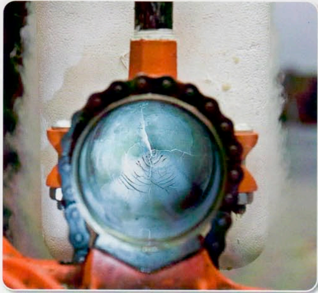
Close-up of a four-inch ice plug under 200 psi.
