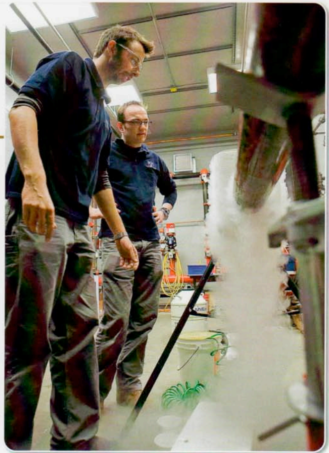
Nitro Pipe freeze in progress.
